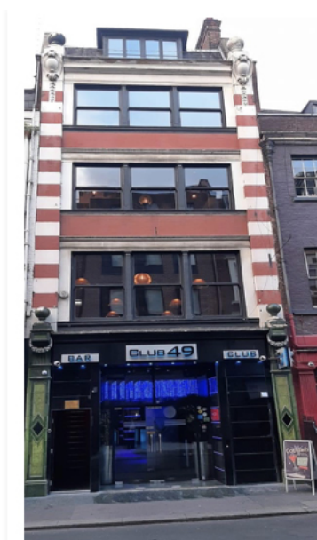
Our building in Greek Street as it is today. The studio was where the small windows at the top can be seen.
